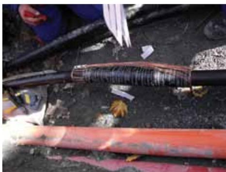
Reconnection of the screen wires before outer sheath restoration is completed
