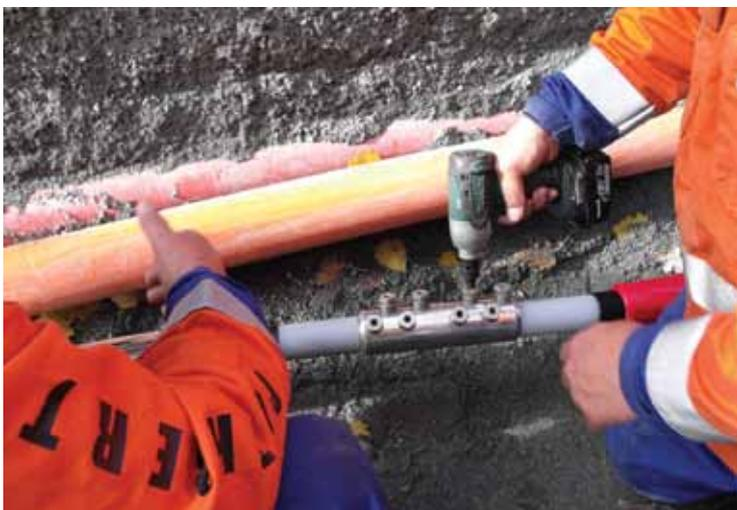
Recently Andrew Wooles along with Bart Foord from Electrix completed nine Nexans cold shrink joints for a new feeder in Warkworth.
